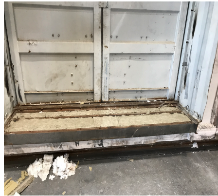
(b) Isolation between the cross members after removing plywood flooring
