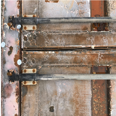
(a) Junction of the door leaves and the header, showing deflection measuring points z_2 , z_5 and z_6
