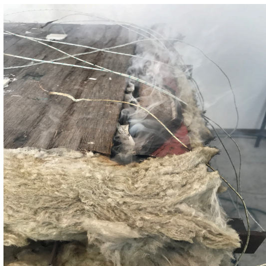
Figure A.8: Smoke at the junction of plywood and steel frame
